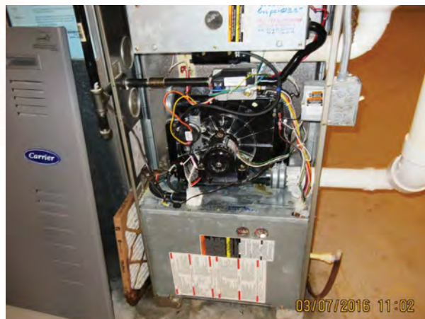
Photo 3. Furnace with minor stains in cabinet.
