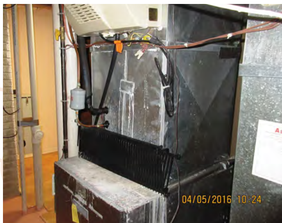
Photo 1. Furnace humidifier leak.
