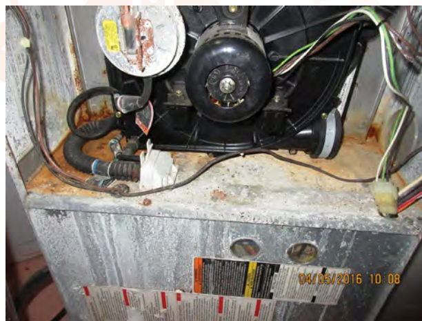
Photo 2. Leak inside furnace cabinet.
