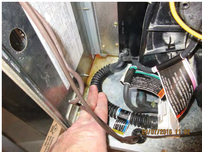
Photo 4. Furnace with water and rust.
